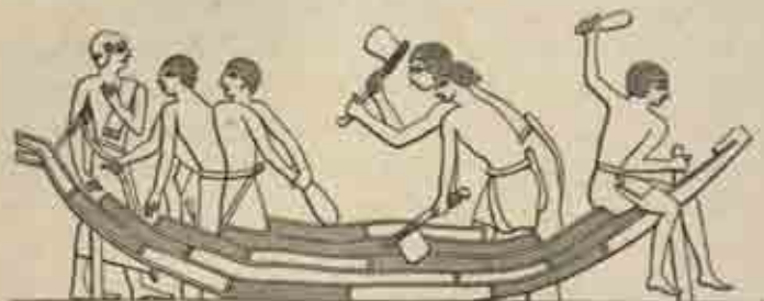
Building a Boat.
